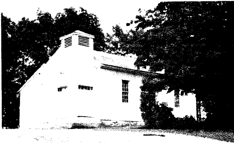
MARSH CREEK CHURCH BEFORE RESTORATION. VESTIBULE AND BELL TOWER WERE ADDED IN ITS GOD'S MISSIONARY DAYS AFTER 1940.
