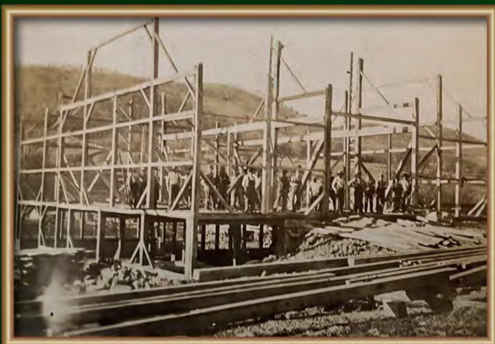
Barn raising, probably at Lee Johnson farm 1924.
